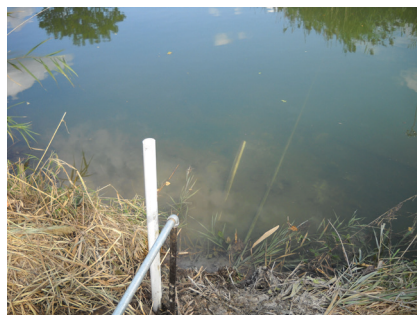
Figure 4. Stilling well and pipe protection of cables.
