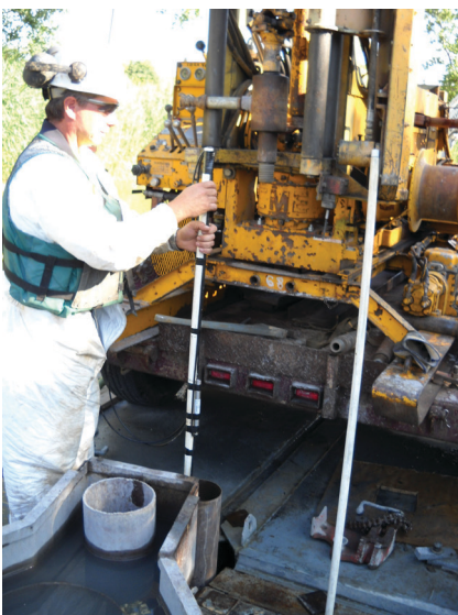
Figure 3. Installation of vibrating wire piezometer and tremie pipe.
