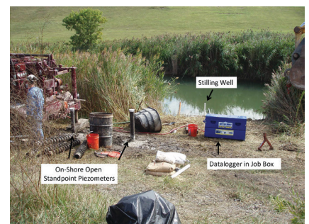
Figure 5. On-shore monitoring location and on-shore open standpipe piezometers.
