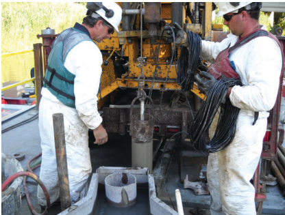
Figure 2. Drill rig on barge.
